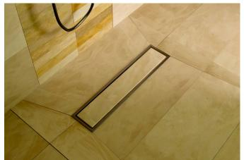
Linear drain—cover filled with tile.
